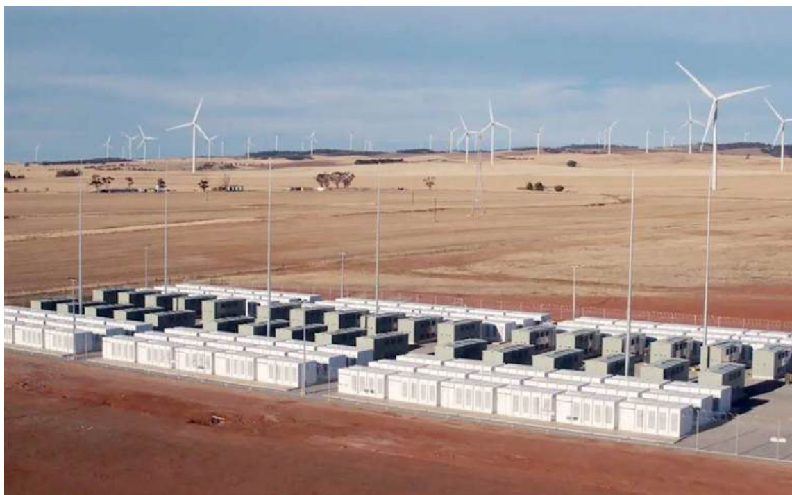
Figure 3-4 Example of a BESS
