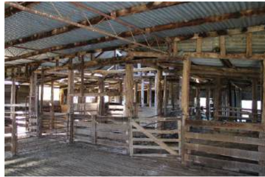
Figure A-21 Internal view through the Waringah Woolshed. Flat roof later addition in the foreground, original section to the rear.
