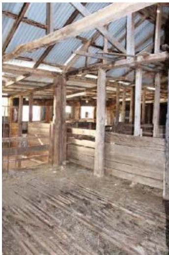
Figure A-22 Looking through the original section of the Waringah Woolshed. Timber floor boards in poor condition.
