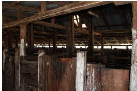
Figure A-18 Shearing pens along the western side of the Woolshed, timber stained with lanolin from shearing activities.
