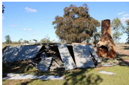
Figure A-25 Collapsed building within the Waringah Homestead group.
