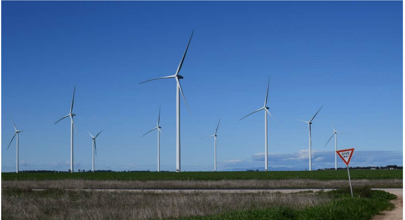
Plate 1 – Typical wind turbines (Senvion 3XM) 211m tip height, Murra Warra VIC (Image: ©GBD Pty Ltd 2022)Plate
